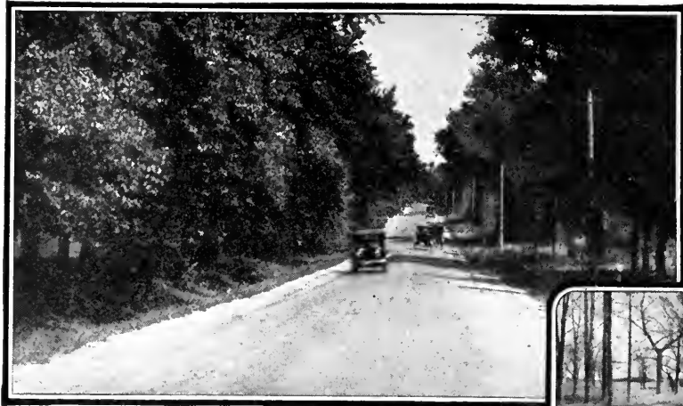
Dundee Road, Elgin Township, Elgin, Ill., gravel macadam maintained with "Tarvia-B"
